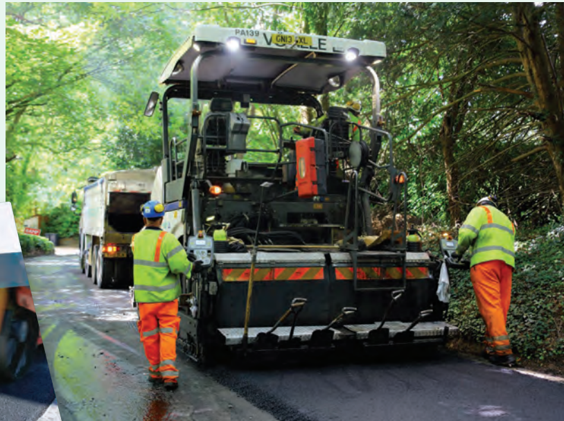
Lower fuel usage and reduced emissions are among the environmental benefits of laying Warm Mix Asphalt
